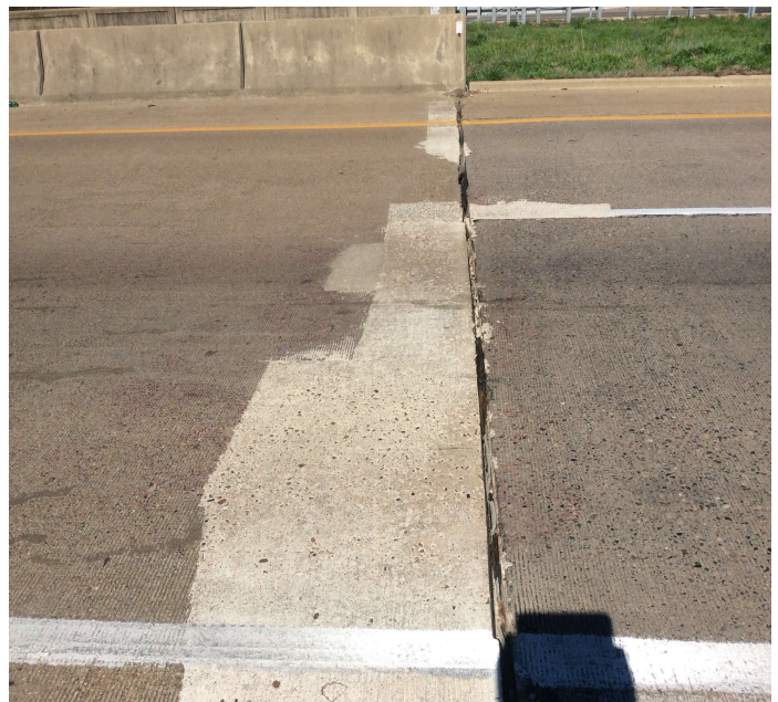
PHOTO 2 Description Joint material missing in joint 8. ....
